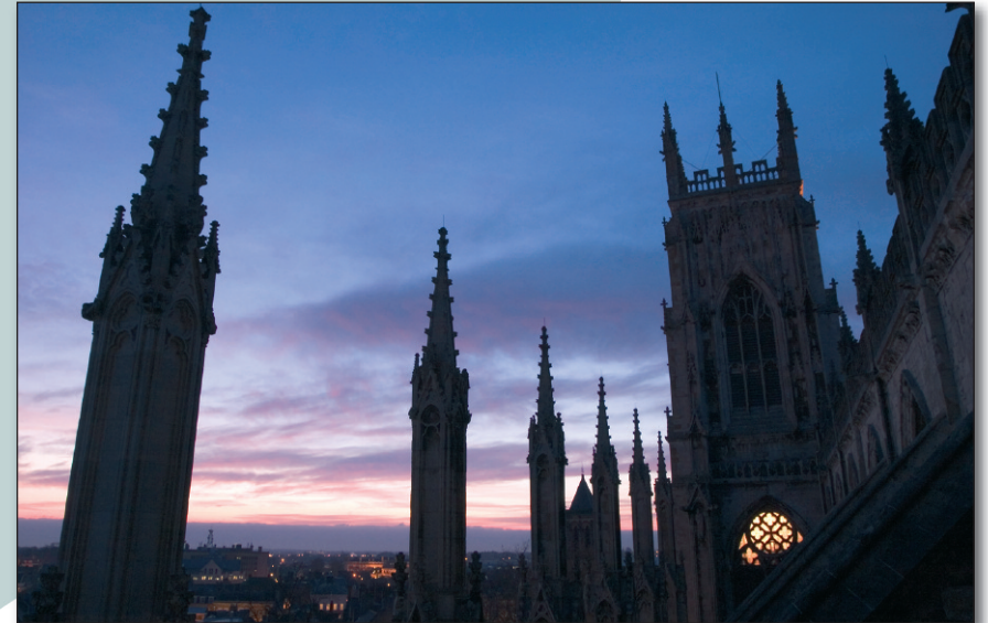
The ornate pinnacles silhouetted against the sunset viewed from the south transept roof which leads to the steep Central Tower steps.
